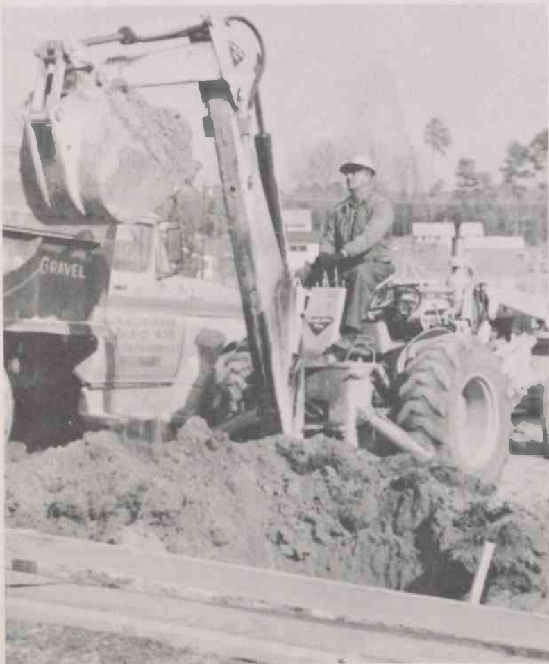
FURTHER GROUND-BREAKING is done by a steamshovel.
