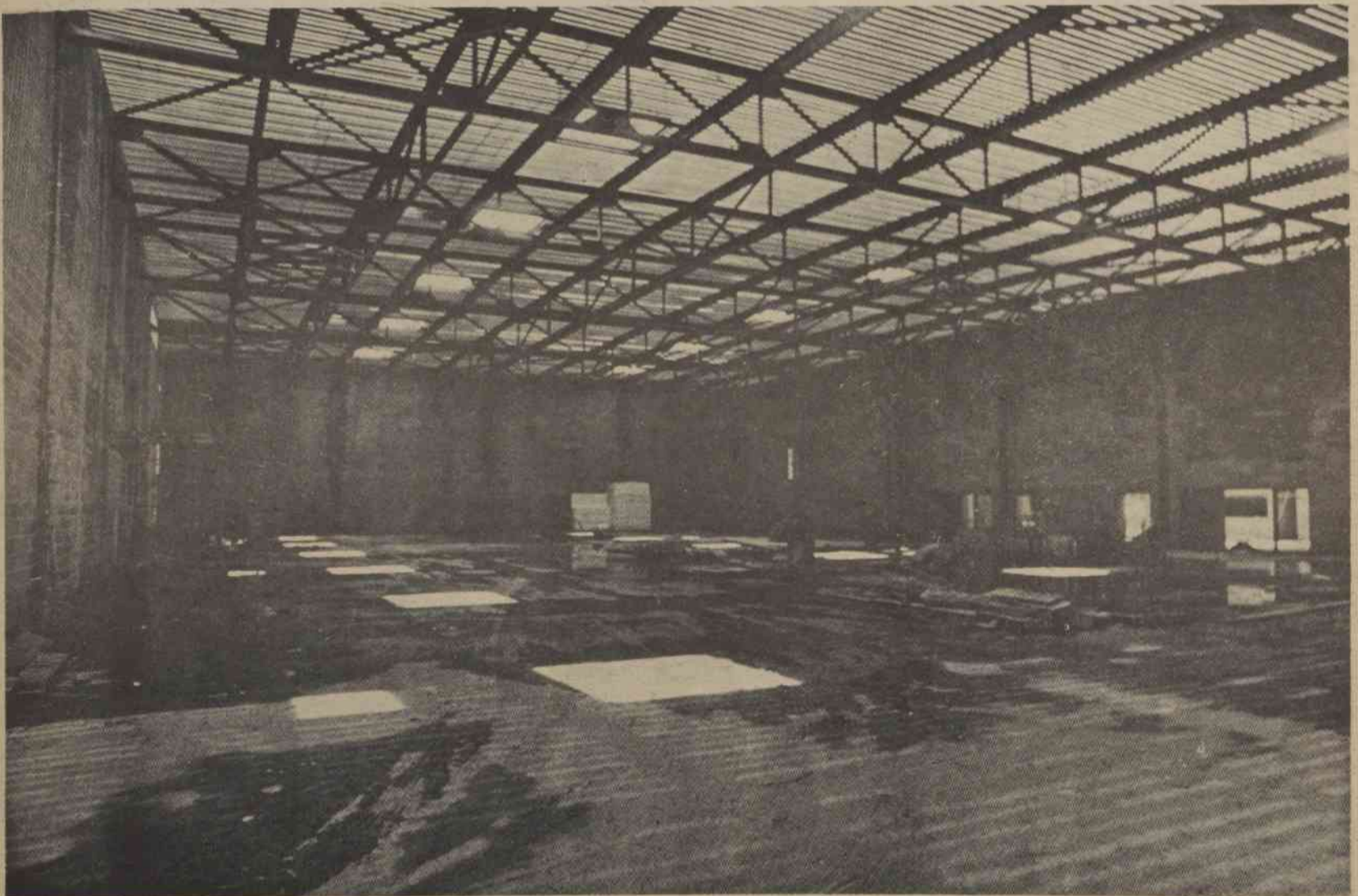
Basketball court area before roofing was completed.
