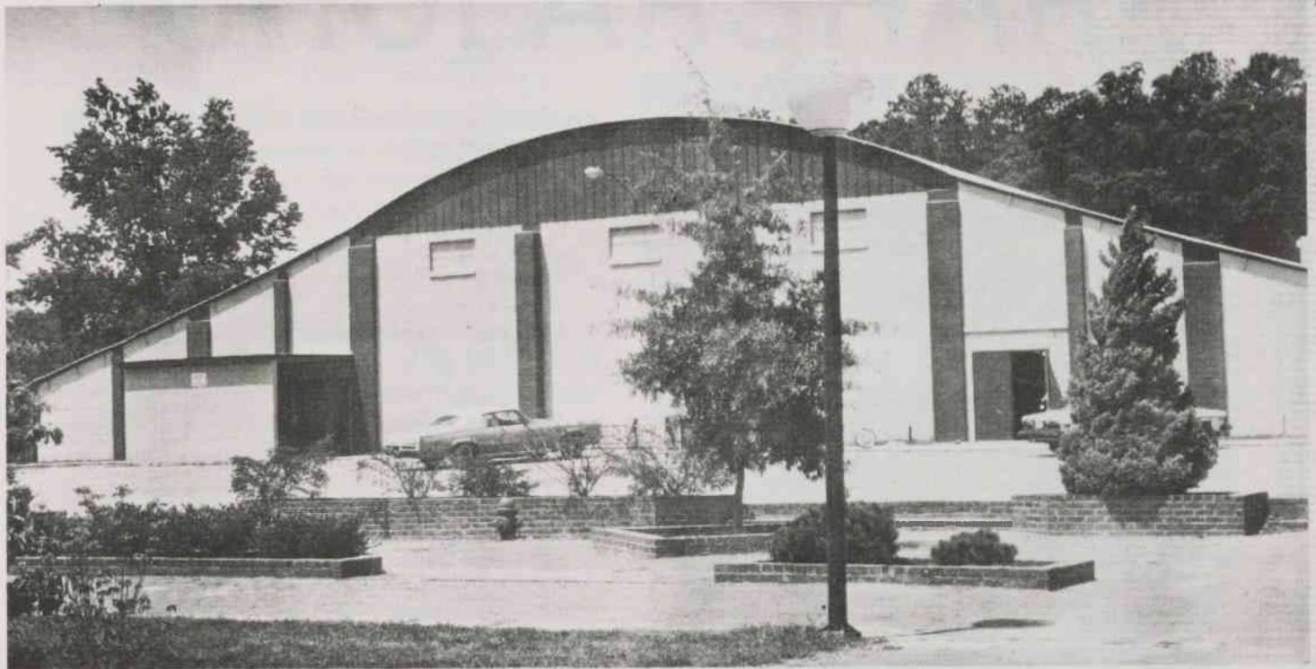
After The old gymnasium takes on a new look as it becomes Lakeside Student Center. An additional entrance has been provided, along with other exterior improvements.
