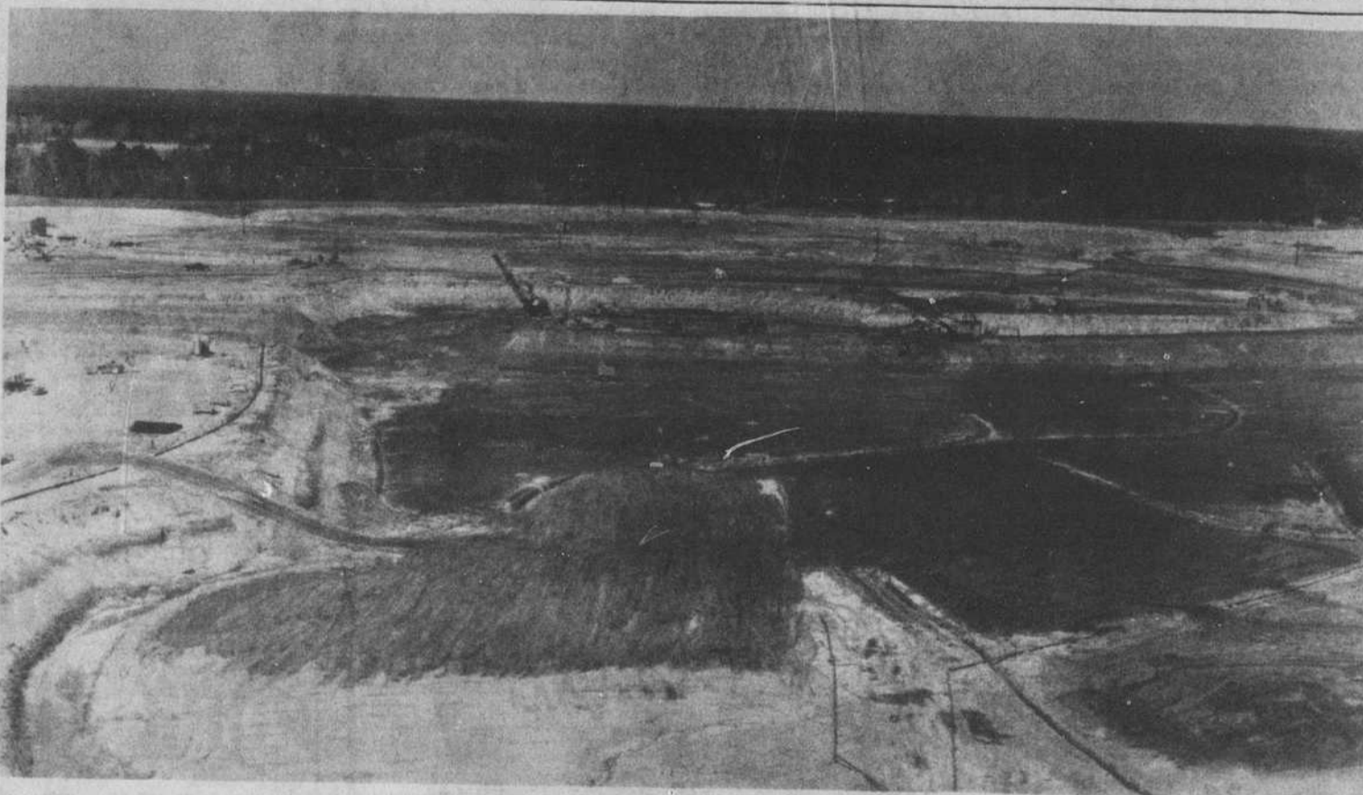
Huge Hole In The Ground
