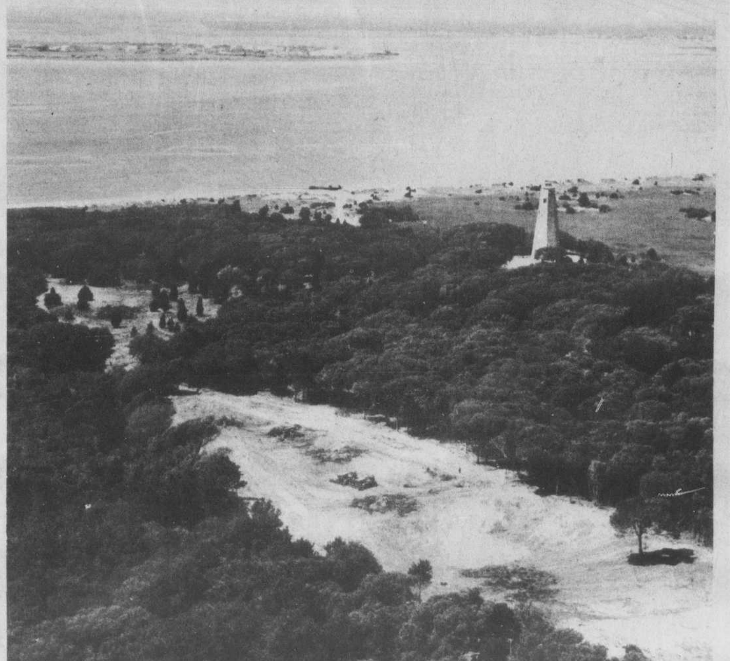
WORK IS WELL UNDERWAY on the 18-hole golf layout at Bald Head Island. This aerial photo by a staff photographer shows the fairway closest to the old lighthouse.
