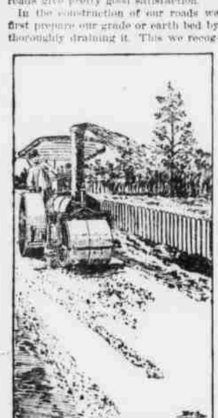
BUILDING A MACADAM ROAD NEAR OAK HARBOR, O.
