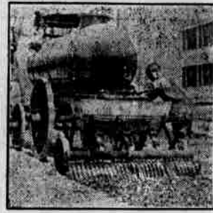
SPRINKLING ASPHALTIC OIL
