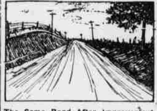
The Same Road After Improvement.
