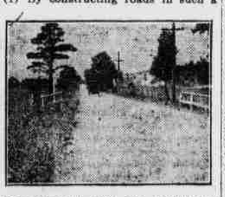
Road Treated With One Application of an Oil Emulsion—Automobile Traveling at Rate of 40 Miles an Hour, With No Dust Resulting.
