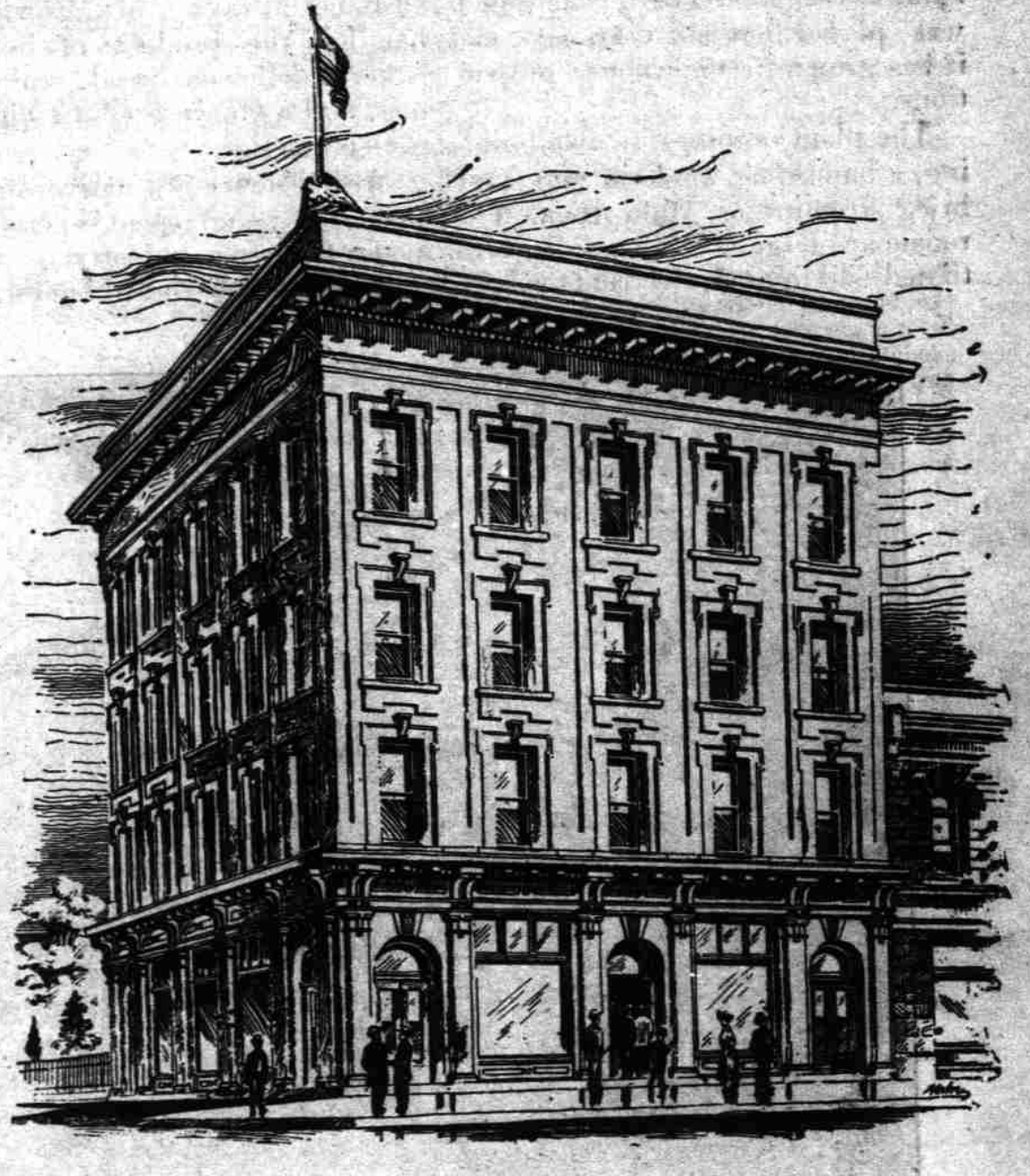
First National Bank Building. (In Course of Erection.)
