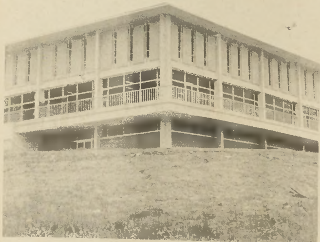
Here Is A Shot Of The Rear Of The Union Addition.
