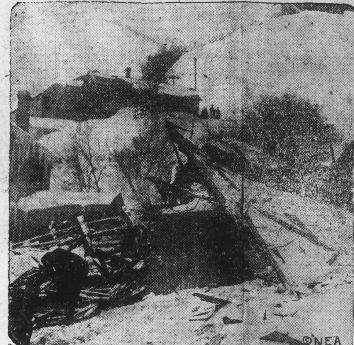
The smashing destruction dealt homes which were in the path of the Sap Gulch, Utah, snowslides again is pictured here. Buildings were crushed to kindling wood as the slides swept down from the mountains which overlook the town. Caught without warning of the disaster, dozens of persons met death or injury.
