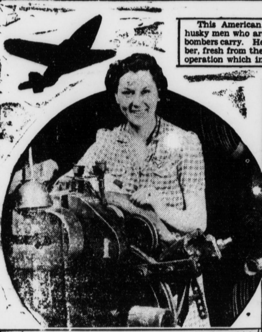
Girls are taking an active part in making the tires which carry General Doolittle's bombing command. Many of them work in the bend room at the General Tire factory. The bend is a steel wire hoop, which reinforces the body of the tire and builds added strength into the finished sidewall. Rubber bands are used in tires for heavy bombers.
