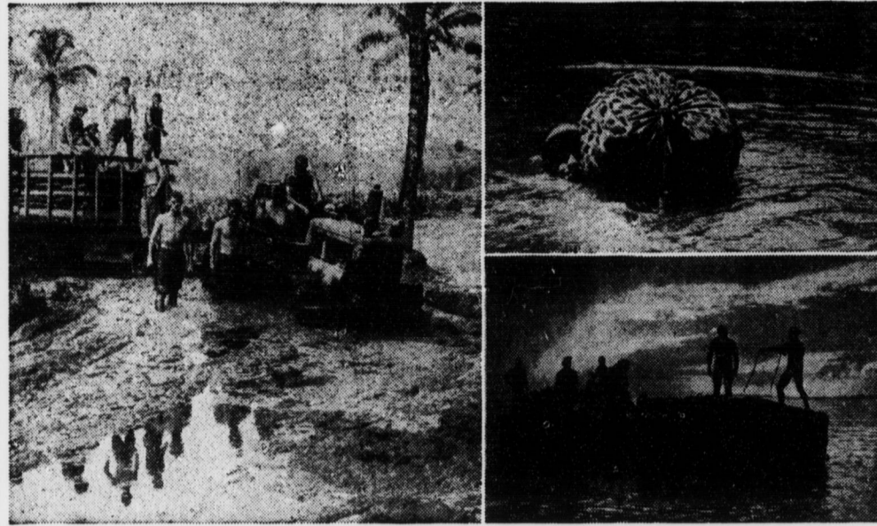
Left: Sandy mud plus daily rainstorms created this type of road for marines during their early days of operation on Bougainville. Jeeps and trucks were unable to get through to front lines until engineers and Seabees surfaced the roads with sea coral. Top right: Pfc. Juan Gonzalez starts across a lagoon in the South Pacific with an inflated poncho or rain cape. Bottom right: Marines work frantically against the setting sun. A whole day's work depended upon their success in getting a tractor raised before dark.
