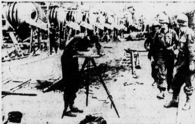
American engineers are shown surveying a 700-foot steel and concrete unfinished ramp in Normandy, which is believed to have been planned for use by the Germans as a launching site for rocket bombs. Assembly line of concrete mixers abandoned by the Nazis are in the background. Not enough and too late was the story of this Nazi effort.
