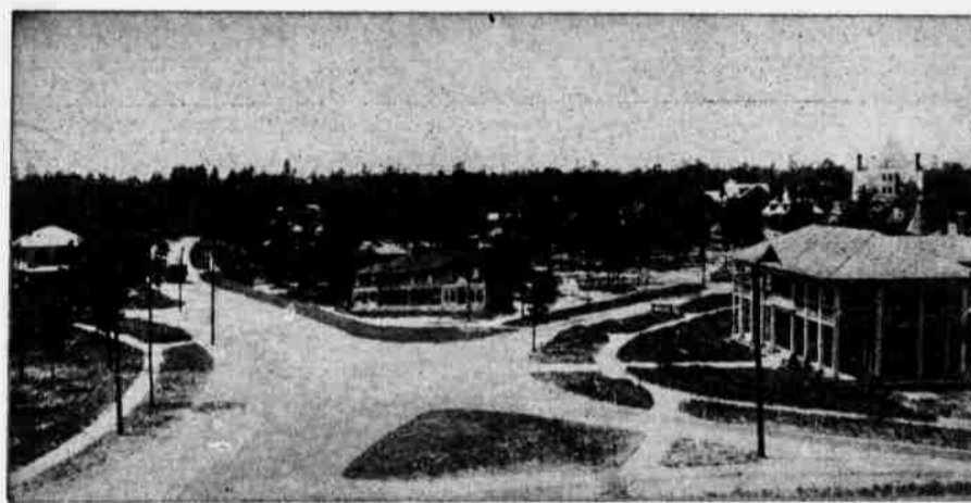
VIEW FROM HOLLY INN, LOOKING WEST.
