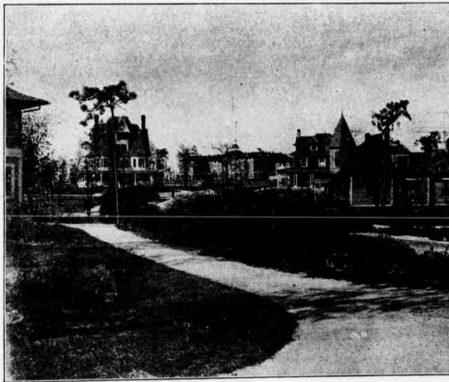
VIEW IN PINEHURST, LOOKING TOWARD THE CAROLINA.
