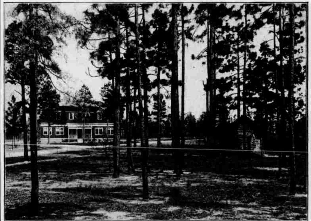
THE SCHOOLHOUSE FROM THE PINE GROVE.
