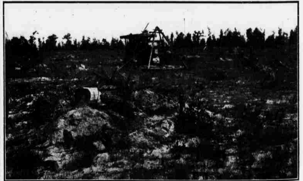
STUMP PULLING ON DROWNING CREEK PLANTATION
