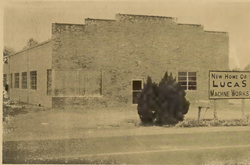
THE NEW HOME OF LUCAS MACHINE WORKS ON U.S. 13 SOUTH OF AHOSKIE
