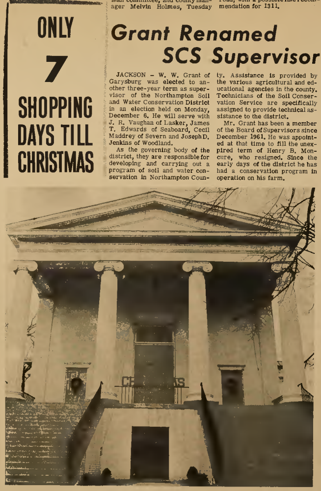
CHRISTMAS GREETINGS FROM COURTHOUSE — The Northampton County Courthouse says Merry Christmas to the people in large red letters above the railing on the second floor porch, flanked by large green wreaths with red bows adorning the heavy wooden doors leading into the court room. Attracting many out-of-county visitors with its architecture, the building's beauty is enhanced during the Christmas season by the traditional decorations.
