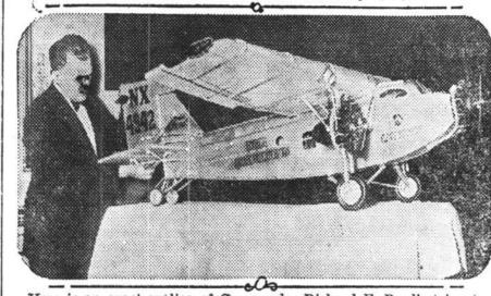
Here is an exact replica of Commander Richard E. Byrd's tri-motor monoplane "Floyd Bennett," built by hand by William Klassen, maitre d'hotel of the Great Northern Hotel, New York City. The plane is built of aluminum and duralumin. It has a swing span of 96 inches, is 66 inches long, weighs 102 pounds and its propellors are powered by tiny motors which revolve them at a speed of 1500 revolutions per minute. The original of that model is now circling over Antarctic wastes.
