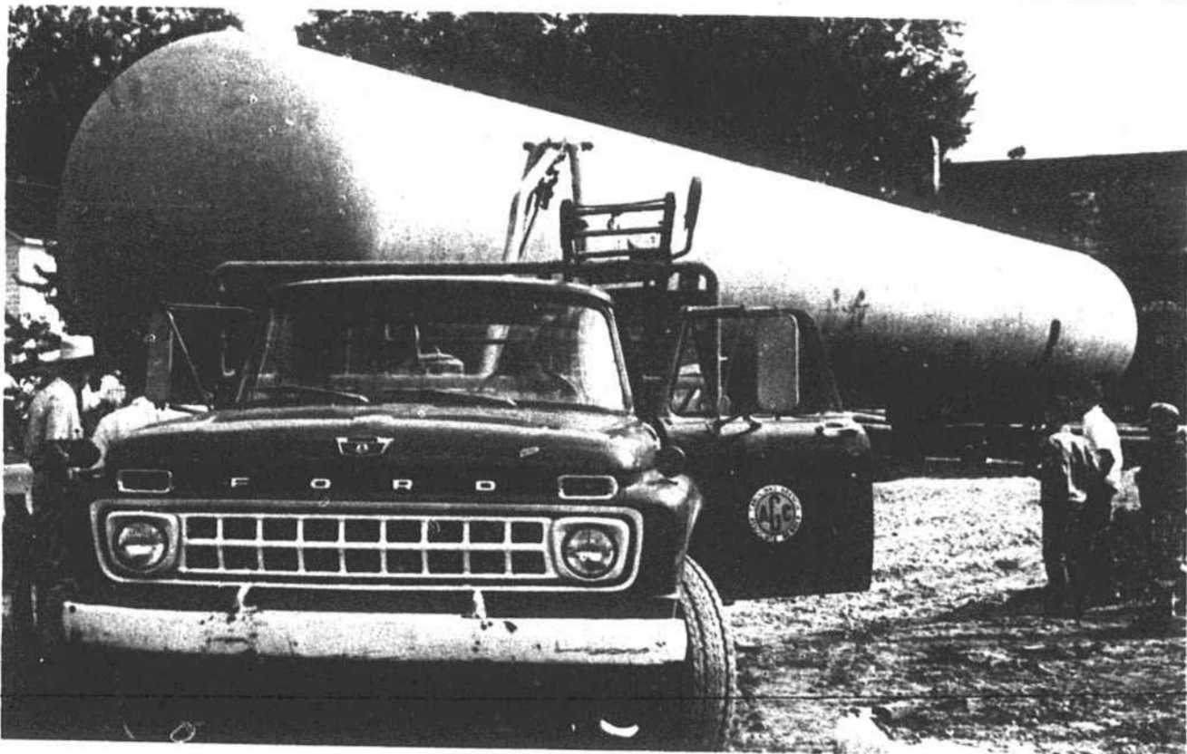
Compression water tank is shown being unloaded at site of old water tank, destroyed by fire, on Tuesday. The 50,000 gallon tank, which is around 90 feet long, was brought to Warrenton from Gastonia by tractor and dolly. Due to its length and in order to avoid heavy traffic the tank was brought
