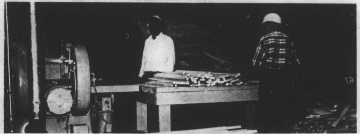
MOLDING PANEL BEHIND RIP SAW.
