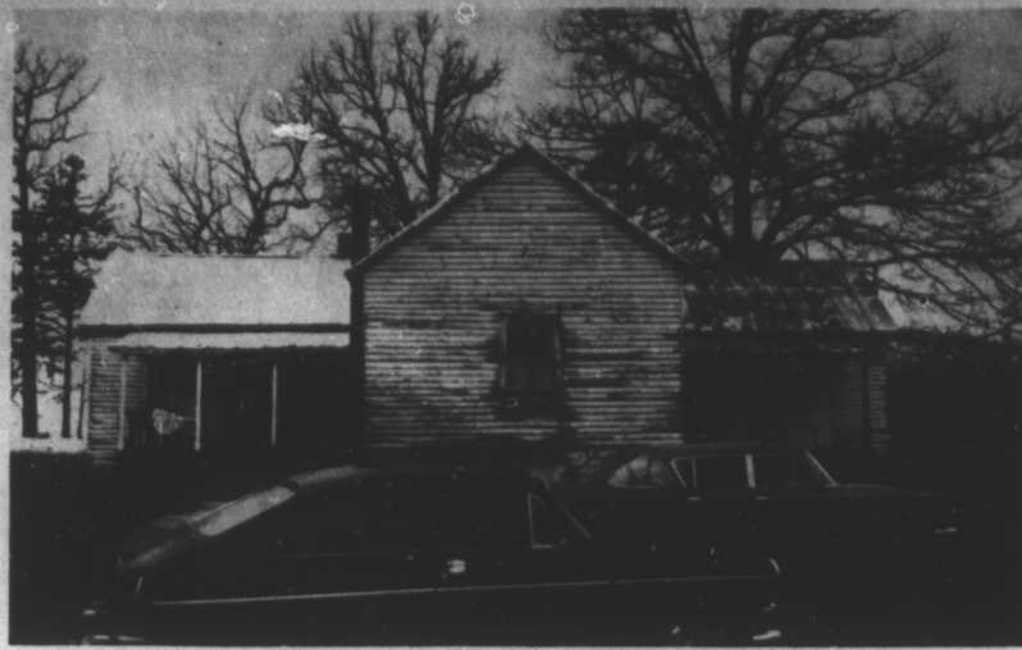
COMMUNITY BUILDING BEFORE PAINTING
