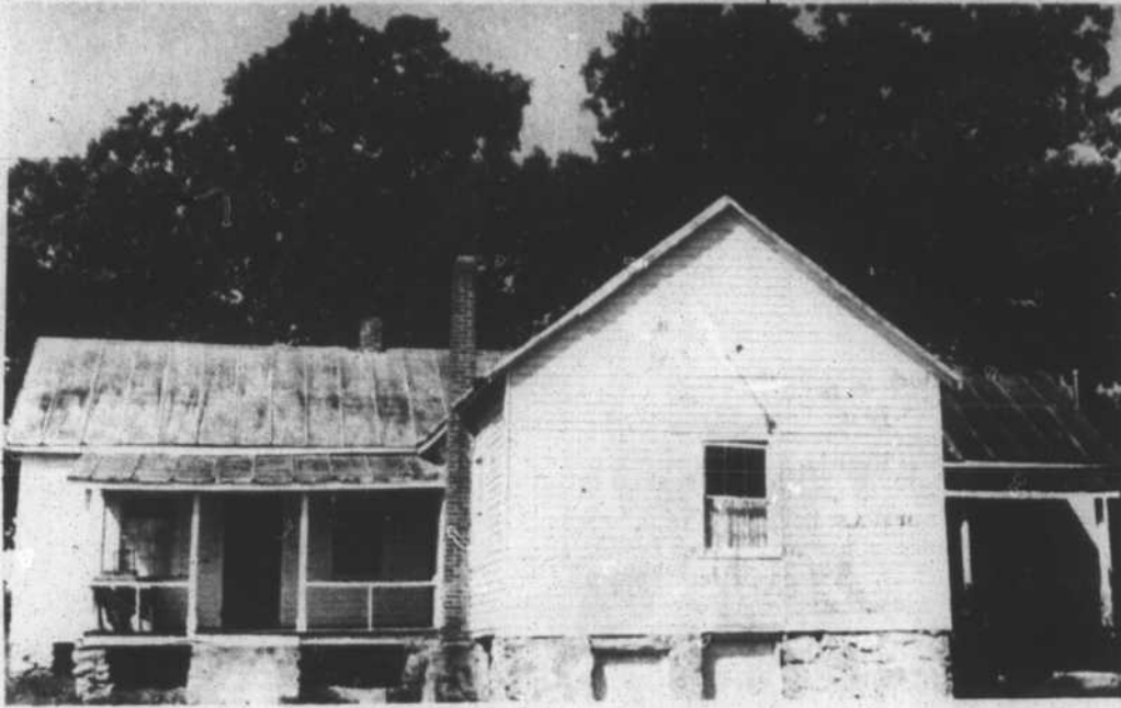
SAME BUILDING AFTER PAINTING
