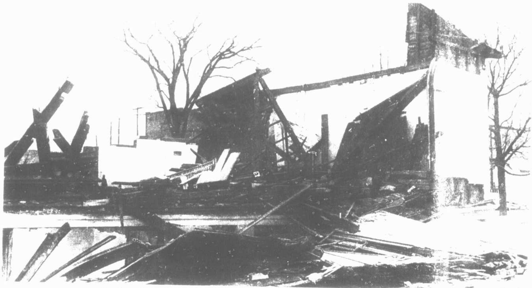
No One Was Injured In Cave-In Of This Old Warrenton Church On Tuesday
