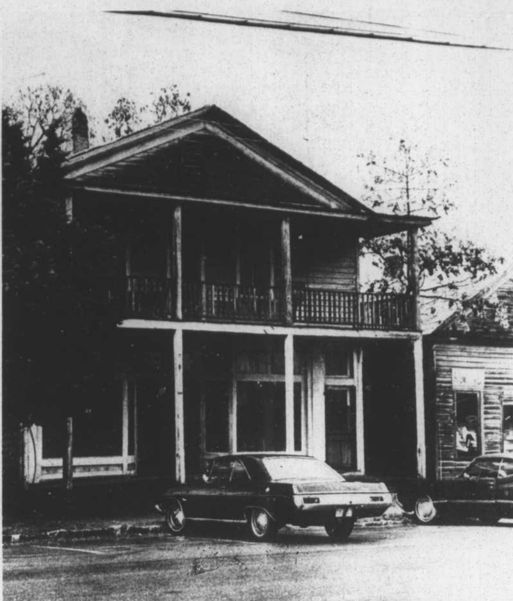
Norlina Board Wants This Old Building Removed
