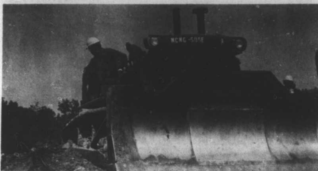
PREPARING QUARRY —Specialist Tony V. Williams operates a bulldozer in readying the site of a quarry furnishing stone which Warrenton and Henderson National Guardsmen are using in their annual training exercise at Butner this week and next. [National Guard Photo]
