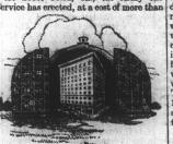
\$2,000,000, a large airship hangar. The we,twt,twt, a large airship hangar. The huge structure could contain a 10-story office building with a 50-foot tower on the roof. The hangar, which is built of steel, concrete, and glass, is 825 feet long and 225 feet high. At the end are large steel doors opened and closed by electric motors that travel on railroad rails.
