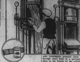
with tremeadous pressure force it through small holes in a perforated plate at the bottom of the cylinder. This is called the "trafila," and its form fixes the character of the product. The hollow form of macaroni is given by a steel pin in the holes. Smaller holes without pins produce the solid spaghetti.
