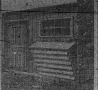
A Shutter for the Poultry House That, While Providing Ample Ventilation, Eliminates Draft, as It Closes Automatically in a Wind.
