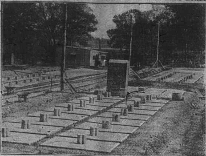
Slabs to Be Tested by Impact Machine—Government Tests to Improve Road Construction.
