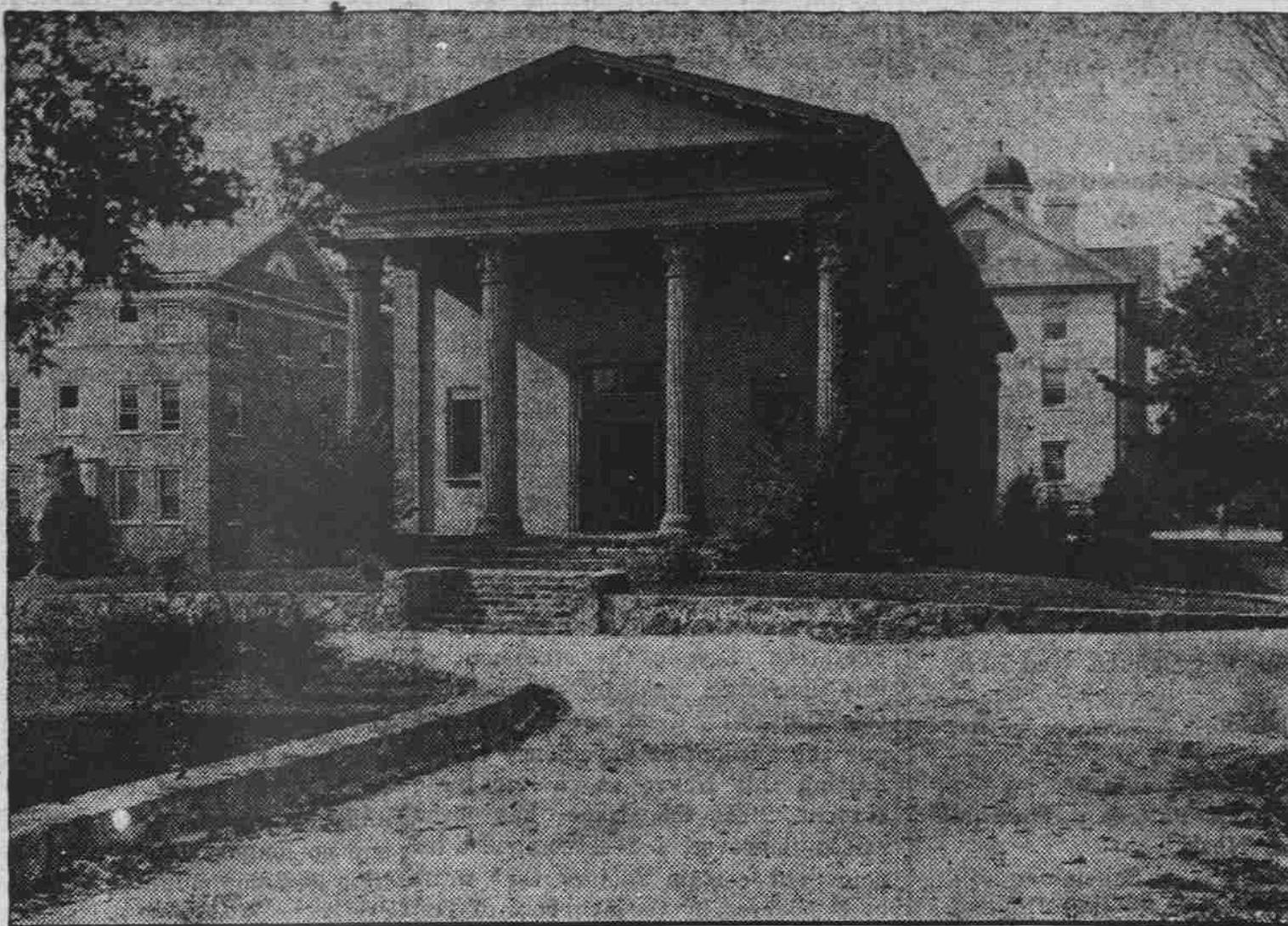
Shown above is the newly-renovated Playmaker theater that was gutted by fire during August of last year. Long a landmark famous for its beauty of structure and as the center of activity for the dramatic arts department, it is going back in service tonight when a group of student-written experimentals will be produced at 7:30 to dedicate its new dress.
