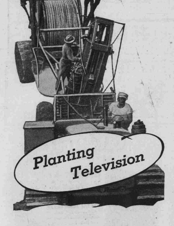
A BOUT 7,000 miles of coaxial cable will be added to A our plant during the next few years. Inside each cable are six or eight copper tubes - each pair a broad communications highway over which two television programs or nearly 500 long distance telephone calls can travel. Giant plow-trains will "plant" much of this cable deep in the ground-safe from storm and fire.
