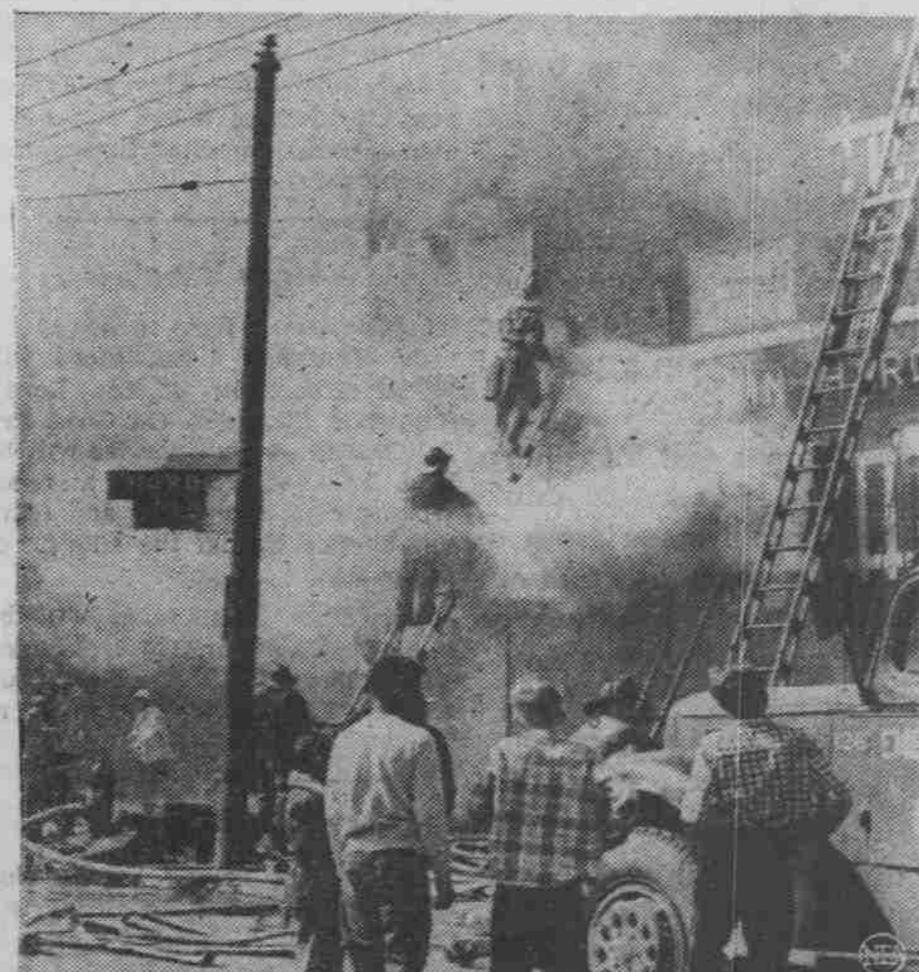
TWO FIREMEN WERE INJURED at this $100,000 blaze which destroyed a two-story commercial building in Kansas City, Mo. Firemen, partially obscured by smoke, climb ladders to battle the spectacular blaze.—NEA Telephoto.
