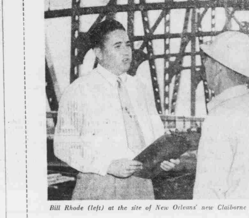
Bill Rhode (left) at the site of New Orleans' new Claiborne Street Industrial Canal Bridge.
