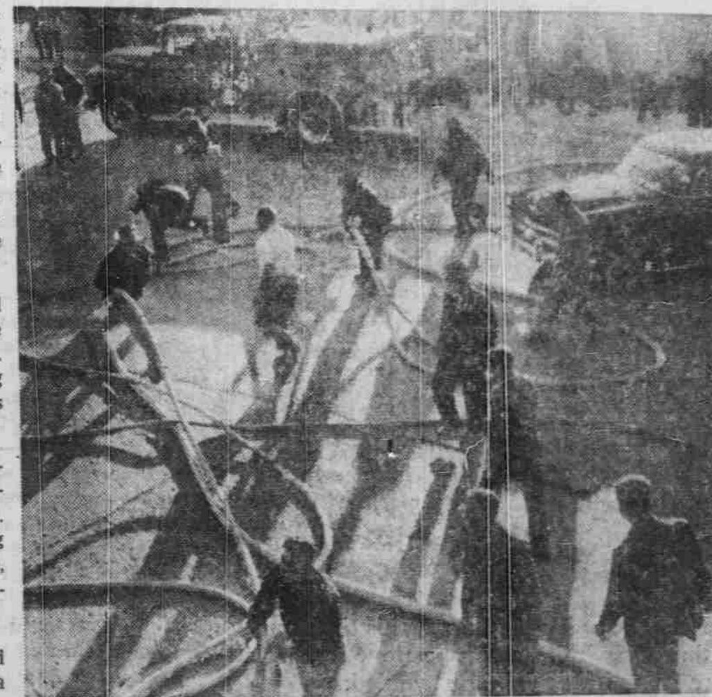
FIRE SCENE —Firemen, volunteers, and spectators are shown with a tangle of fire hose as they work to extinguish the fire which gutted part of the University storeroom yesterday morning.
