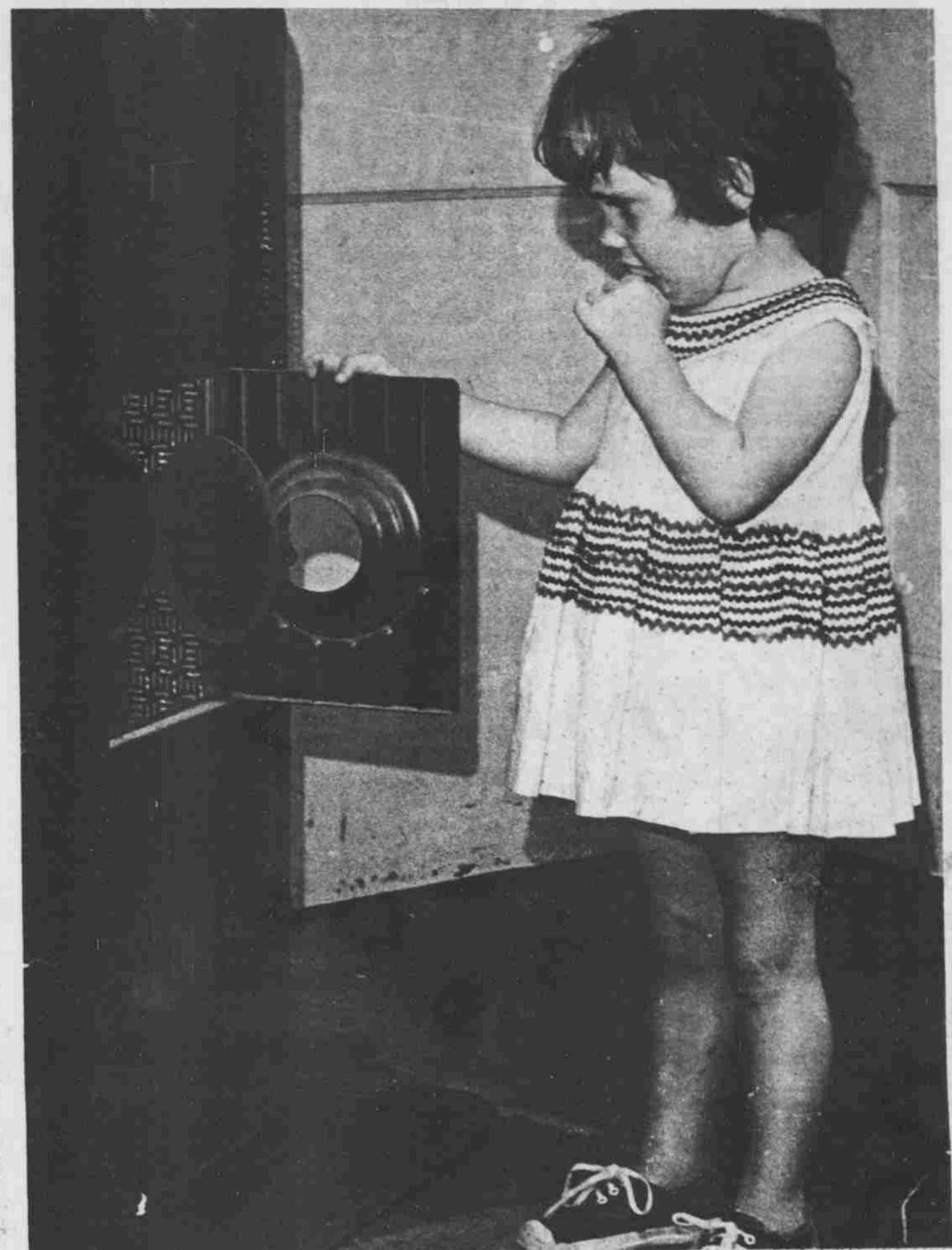
DANGER —Three-year-old Lawson Barber, herself a resident of Victory Village, demonstrates the way to use the kerosene space heaters in Village Apartments. The main thing to do, she says is be careful! Heaters such as these are the main threat to fire safety in the Village according to the University Rental
