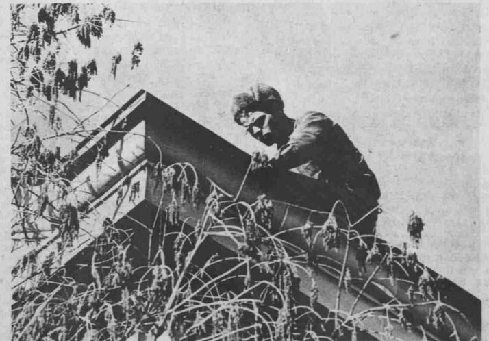
On the Corner of South Building's roof, a workman repairs the tin guttering.
