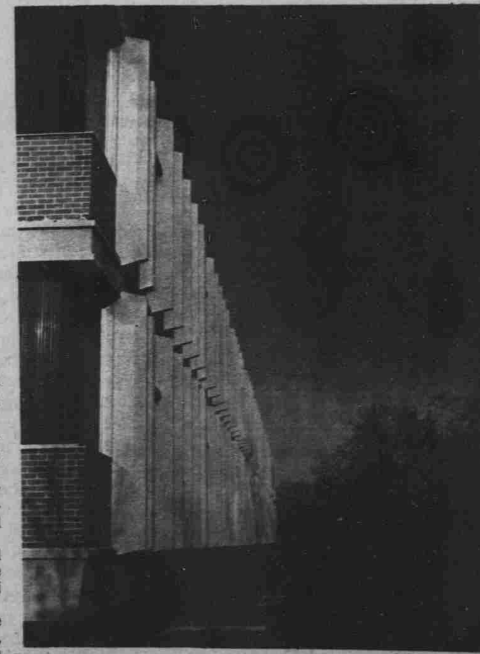
Last spring the DTH ran a picture of workmen finishing up work on Davie Hall Annex. Now they're done—windows have been put in, most of the walks have been paved and students are attending classes in the Rat Palace
