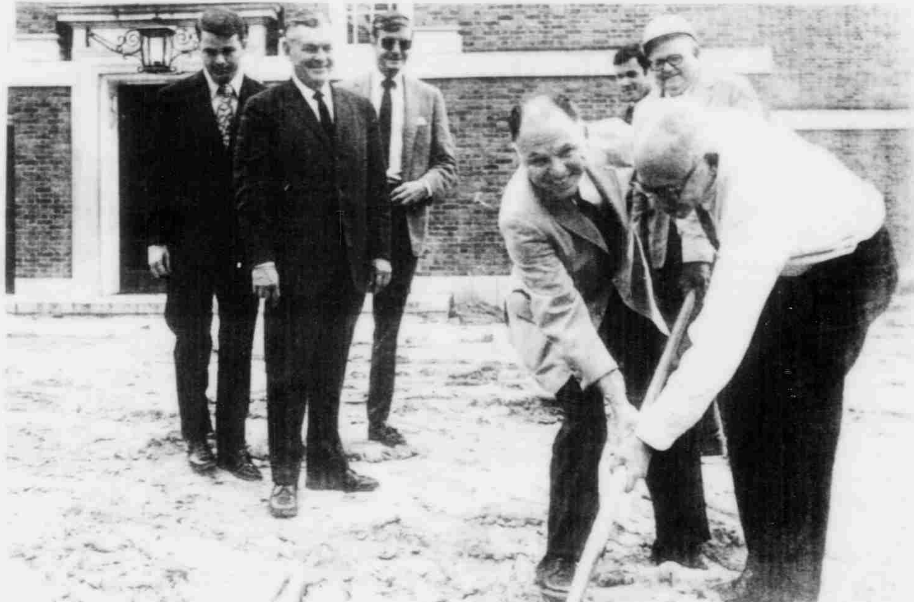
UNC Chancellor J. Carlyle Sitterson (left foreground) and Hugh Chatham, chairman of the UNC Trustee Foundation, hefted a shovel Tuesday during ground breaking ceremonies for the planned addition to the Morehead Planetarium. (Staff photo by Leslie Todd)
