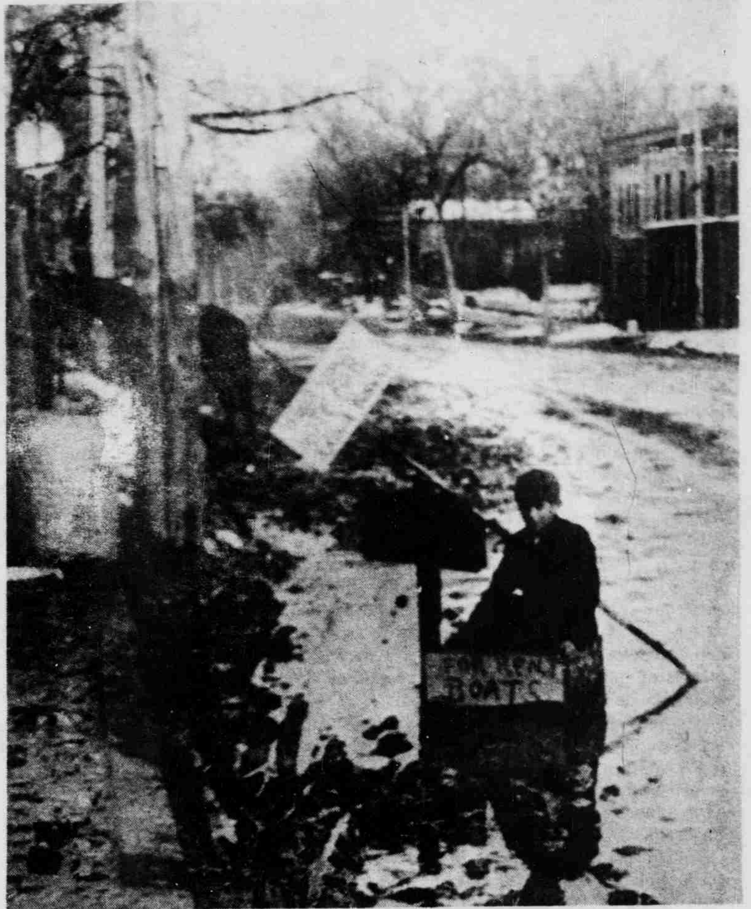
Drainage has always been a problem.
