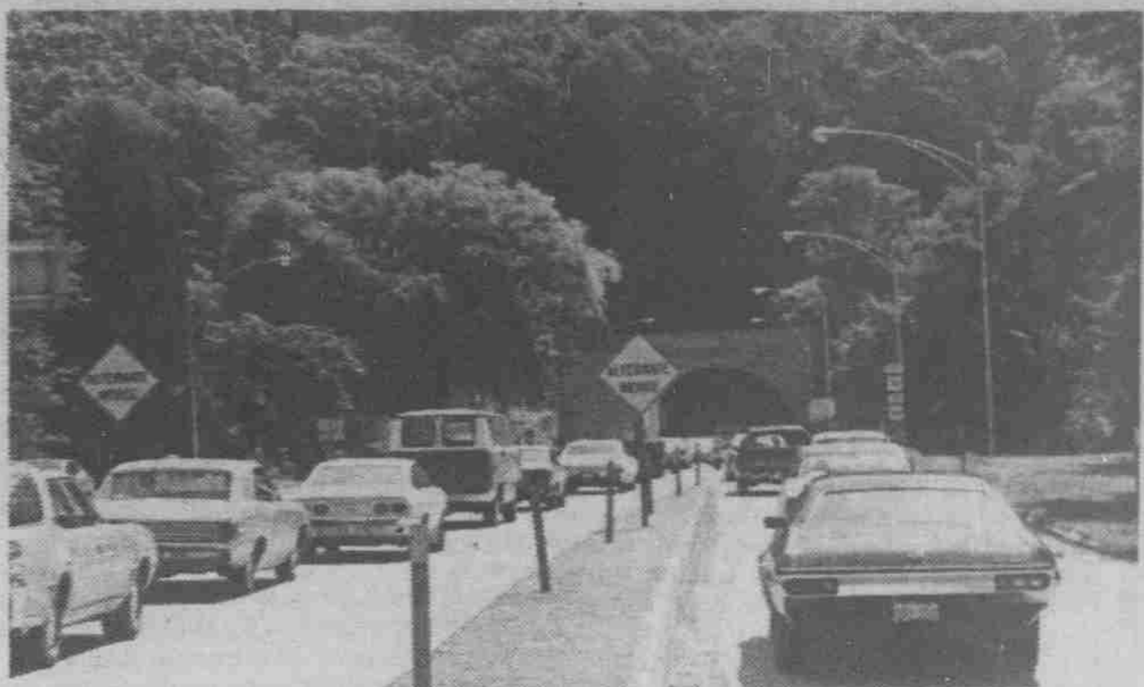
A traffic bottleneck in downtown Asheville, Beaucatcher Mountain Tunnel has created a 15-year-old controversy.
