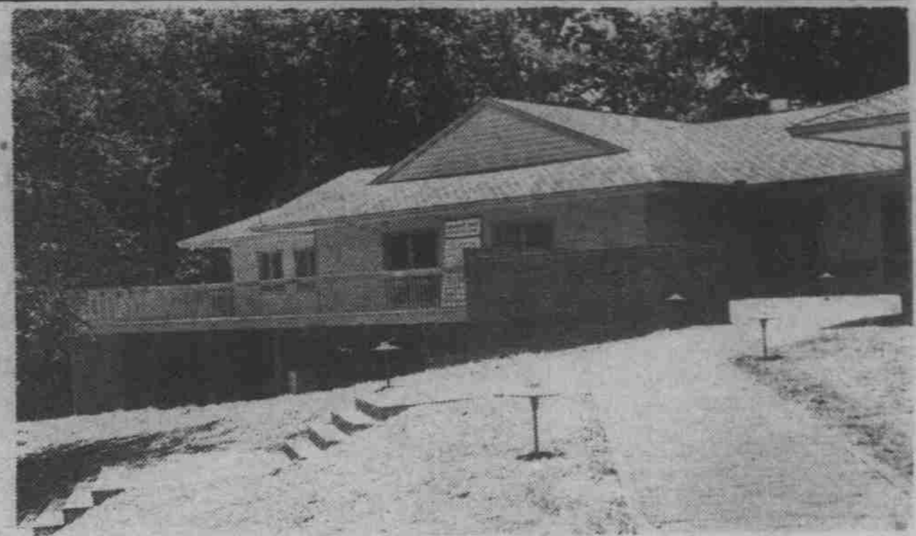
New UNC Press building on Boundary Street ... move planned for next week Photo by Jack Mohr
