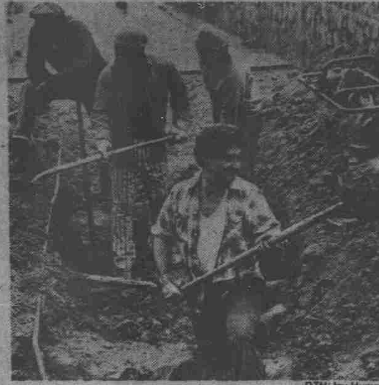
Workers repair leaky pipeline ... ground near libraries caved in
