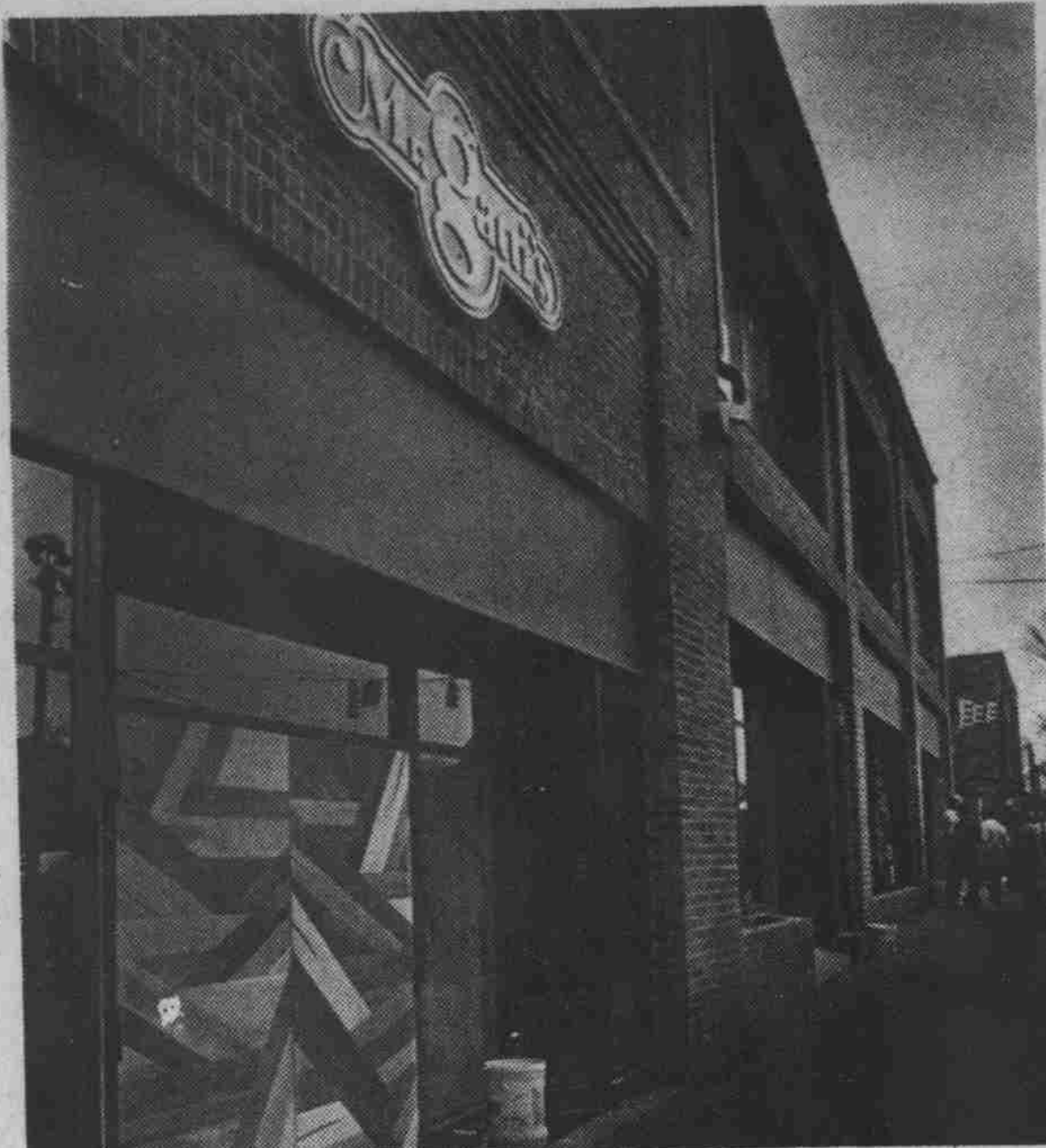
Franklin and Columbia streets' construction nears completion ... old and new businesses will operate in the building
