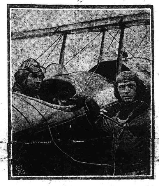
This photograph shows an airplane equipped with the new wireless telephone ready to give a demonstration for government officials at Billing Field, near Washington, D. C. This wonderful apparatus makes it possible to direct the flight of a plane from the ground and for aviators to communicate with each other while in flight. The helmet and mouthpiece are worn in such a manner that sending and receiving messages while piloting a machine is easy.
