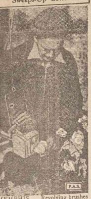
MEMPHIS ... Revolving brushes pull cotton from the boll which is then vacuumed through a large tube to a collecting bag, is the working idea of the newest me-chanical cotton picker now being introduced by its inventor, L. C. Stukenborg. It is claimed the Stukenborg. It is claimed the machine will pick more cotton than two men, and pick cleaner.
