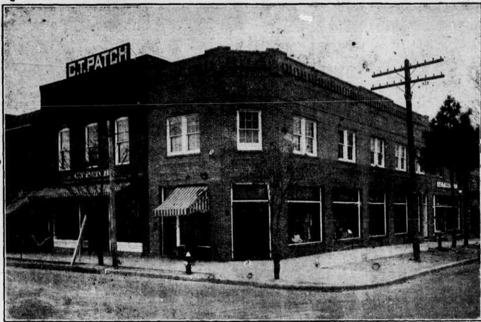
The C. T. Patch Department Store in Southern Pines.
