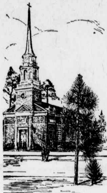
Architect's Sketch of Brownson Memorial Presbyterian Church, Now Under Construction
